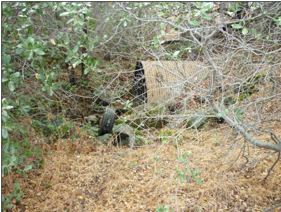
Photo 4. Eastbound I-80 at Sucker Ravine
