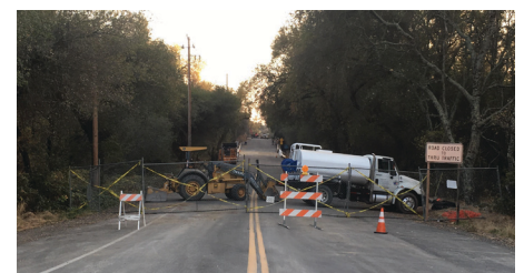
- Replacement of a storm-destroyed culvert and bridge on Penryn Road.
