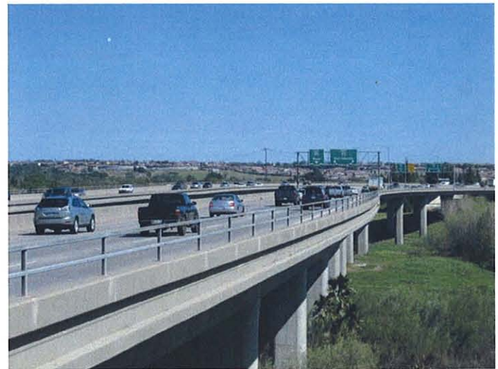
On southbound SR 65 looking south towards the East Roseville Viaduct.
