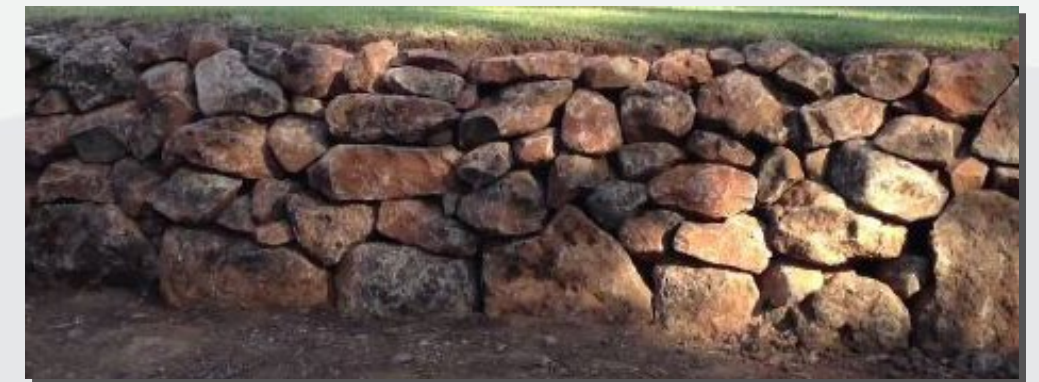
SIERRA BOULDER (ROCKERY WALLS)
