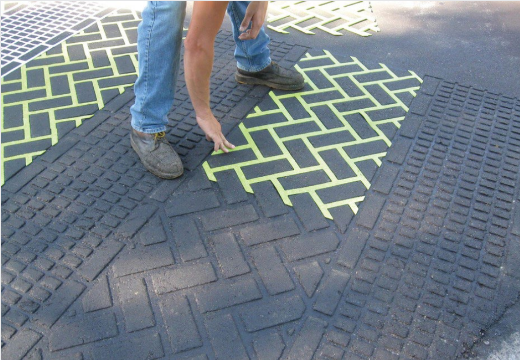
STAMPED PAVEMENT PROCESS: STAMPED ASPHALT CONCRETE (IMPRESSED) WITH INLAID THERMOPLASTIC COLOR ACCENTUATION (CROSSWALKS AND GORE) CUSTOM BASKETRY PATTERN TO BE APPLIED ON ENHANCED PAVING AREAS (CROSSWALKS & GORE POINTS)
