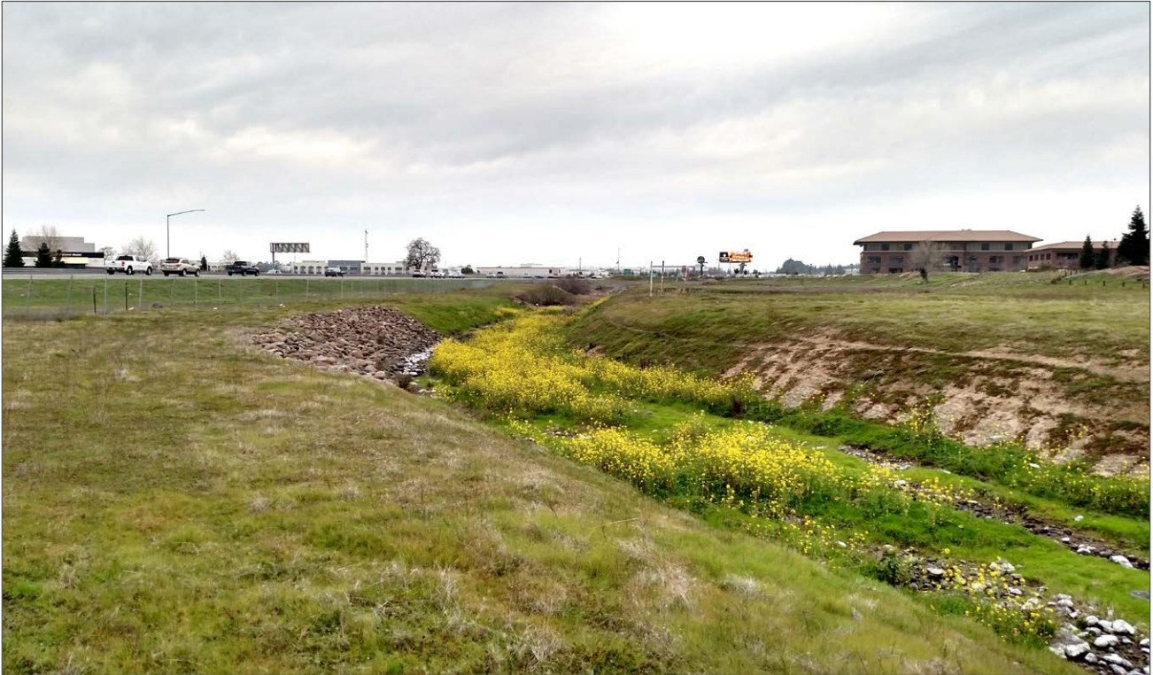
Photo 6: Excavated channel with emergent wetland vegetation along northbound SR 65 north of Blue Oaks Boulevard (facing north; 2/05/2015)
