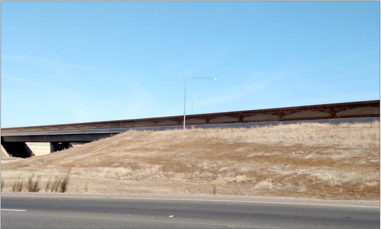
Photo 1: Disturbed area along onramp to southbound SR 65 from Industrial Boulevard (facing northwest; 11/06/2015)
