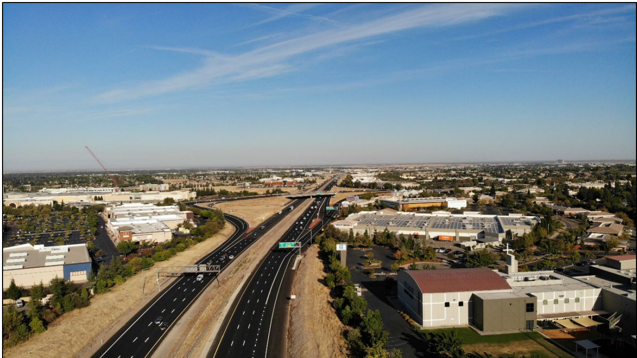
Figure 1: I-80/SR-65 Interchange Phase 1
