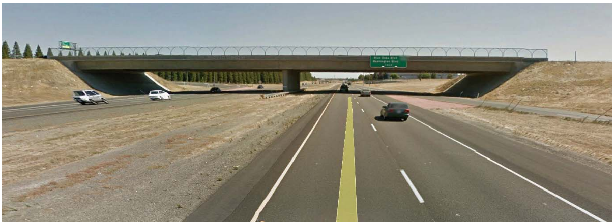
Sunset Boulevard Overcrossing, Looking South
