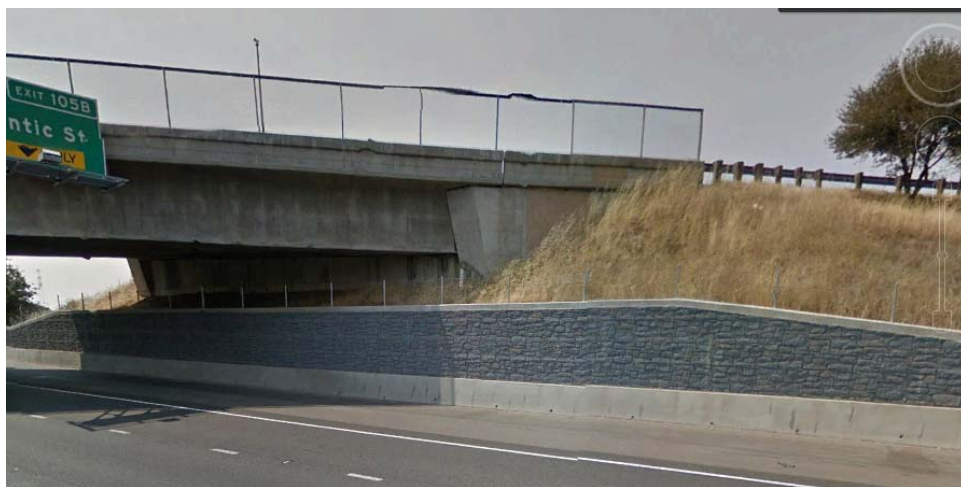
Ground Anchor Texture on Taylor Road Overcrossing on I-80
