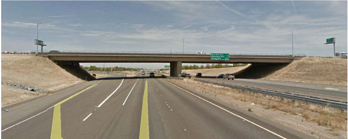
Pleasant Grove Boulevard Overcrossing, looking North
