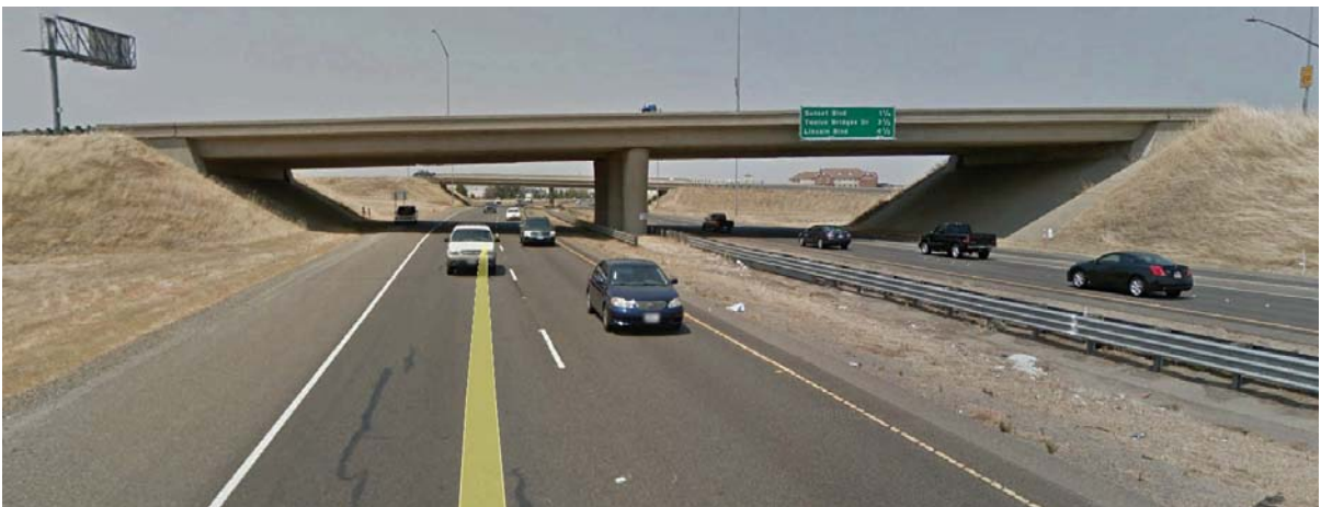
Blue Oaks Boulevard Overcrossing, looking North
