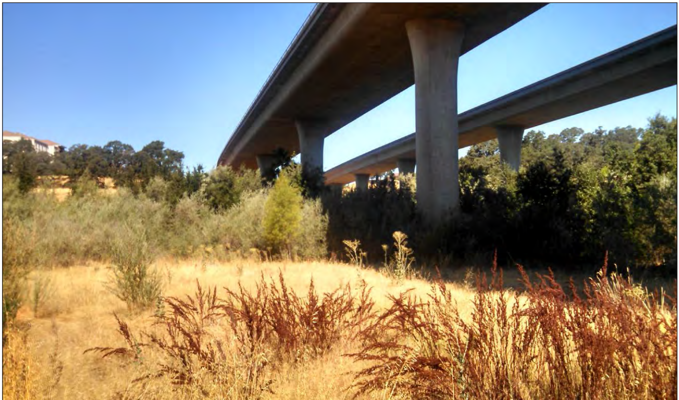
Photo 10: Annual grassland and riparian forest/shrub wetland south of Antelope Creek below the East Roseville Viaduct (facing west; 7/23/14)
