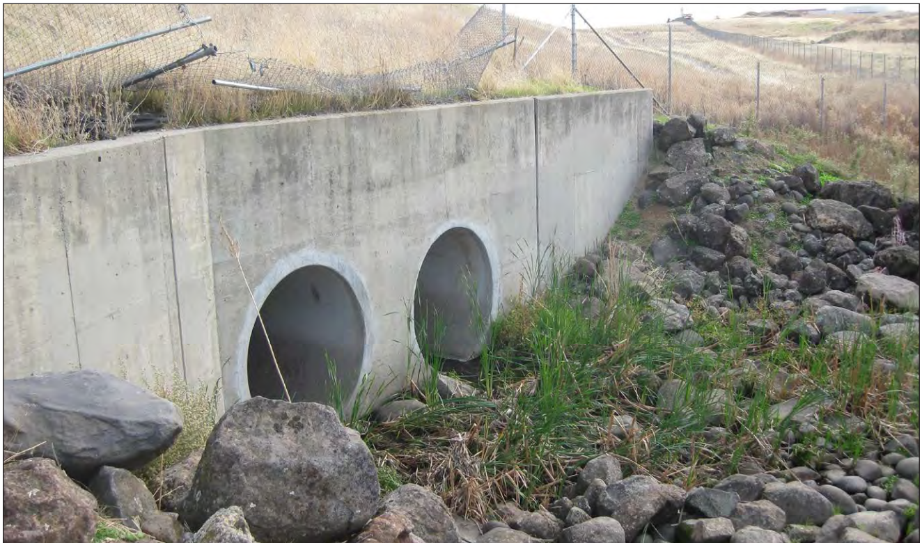
Photo 20: Highland Ravine Culvert on south side of SR 65 (facing southeast; 11/15/12)
