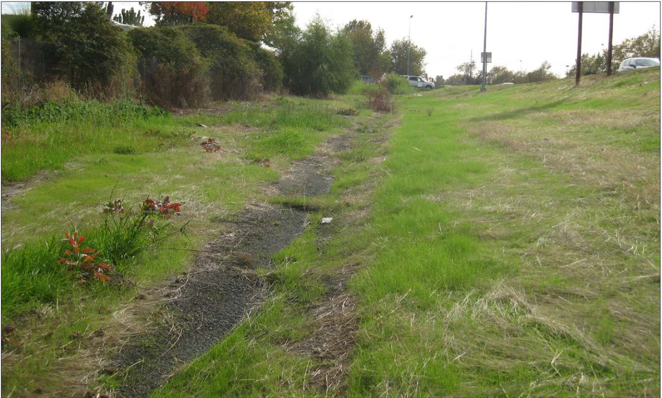
Photo 6: Lined Stormwater Ditch (Facing Southeast).
