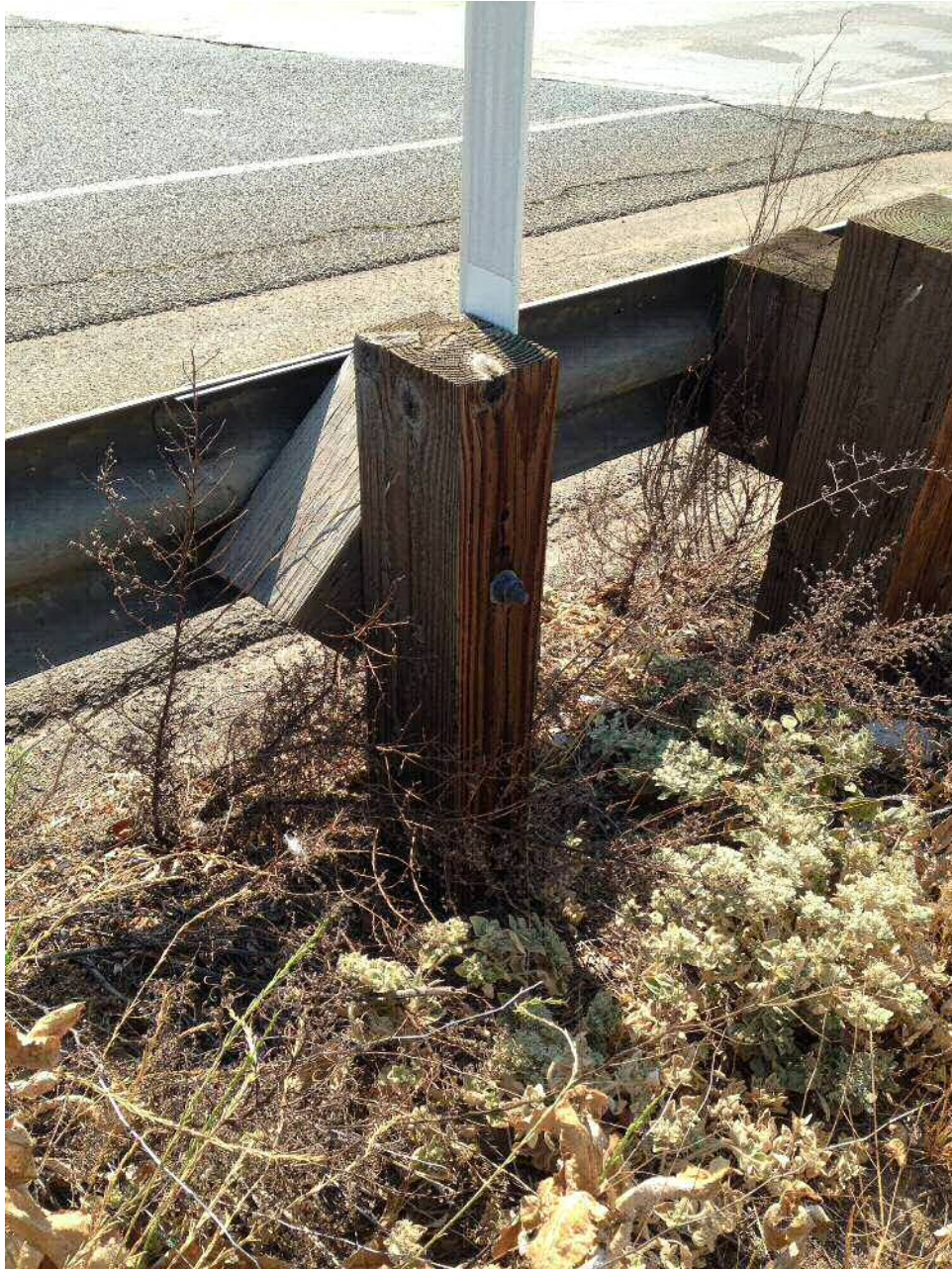
Railing support along roadway
