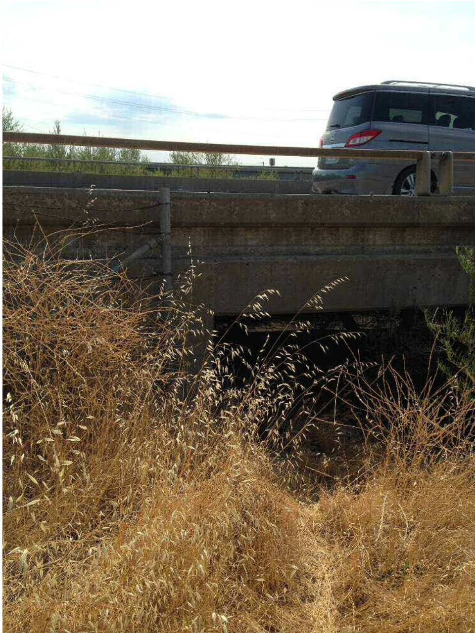
West edge of bridge
