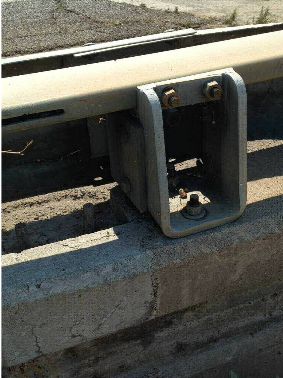
Bridge railing support along bridge
