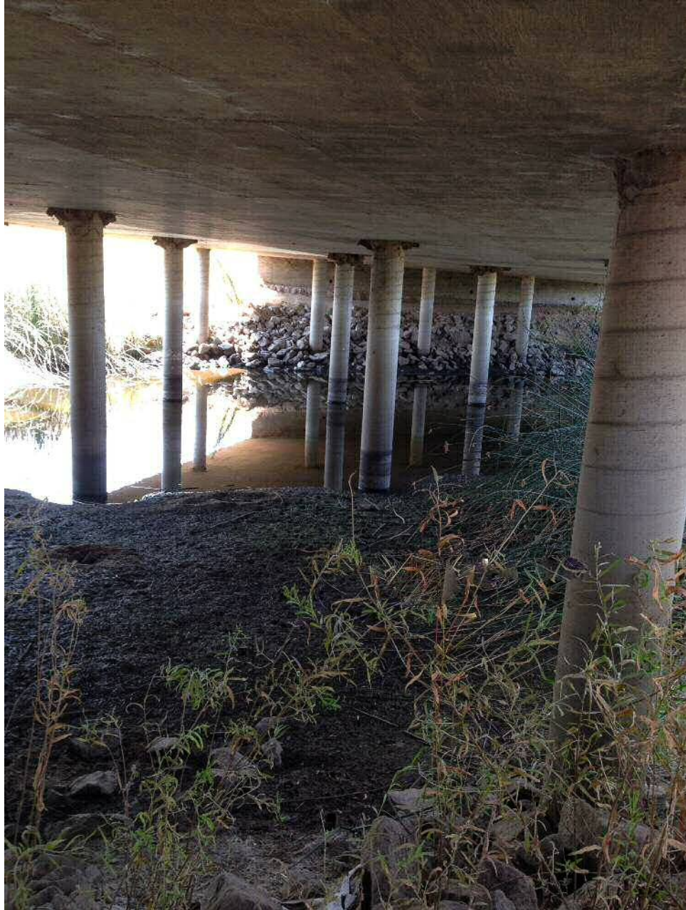
Underside of bridge deck and support columns
