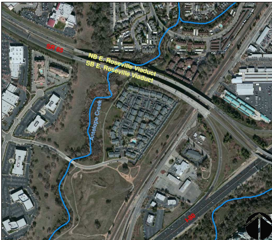
Figure 12. Existing East Roseville Viaduct Bridge at Antelope Creek
