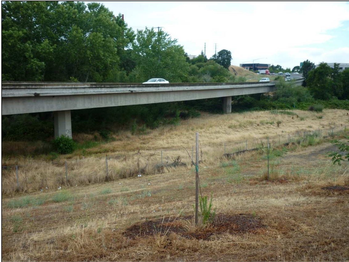
Photo 5. I-80 Off-Ramp to Eureka Road Bridge at Miners Ravine
