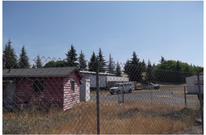
Photo 10: APN 015-162-007 Stonehouse Road office, POD crate and storage building
