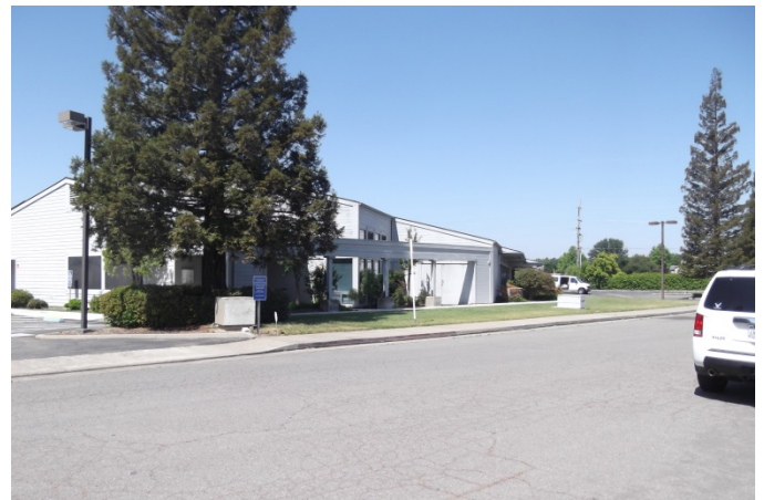
Photo 6: APN 015-162-006 100 Stonehouse Road – vacant offices
