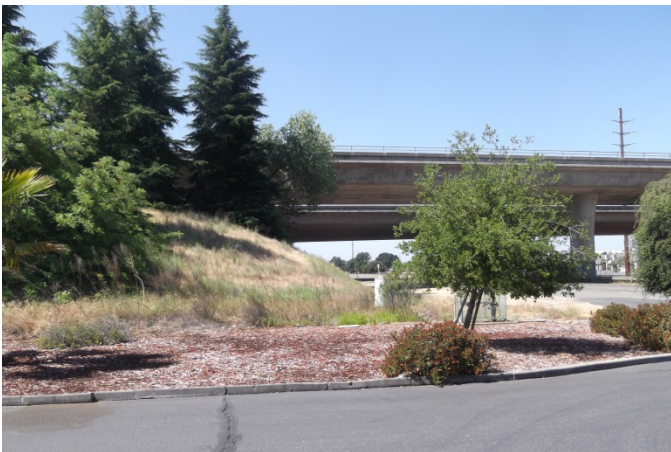
Photo 3: SR-65 overpass at Taylor Road
